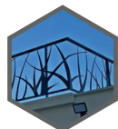
GARDE CORPS PUBLIC
