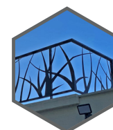
GARDE CORPS PUBLIC
